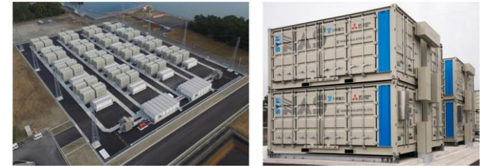
Energy-storage system installed in 2016 -50 MW output -300 MWh rated capacity
