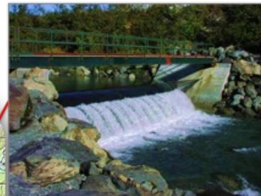
Power Creek Hydroelectric 6248kW (2 x 3124 kW) 25 kV transmission ties to Eyak Substation, Inflatable dams
