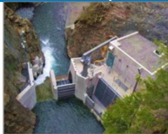
Humpback Creek Hydroelectric Plant 1250kW (2 x 500 kW + 1 x 250 kW) 17,000 foot UG and submarine transmission line
