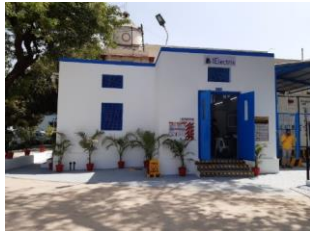
Renovated secondary substation
