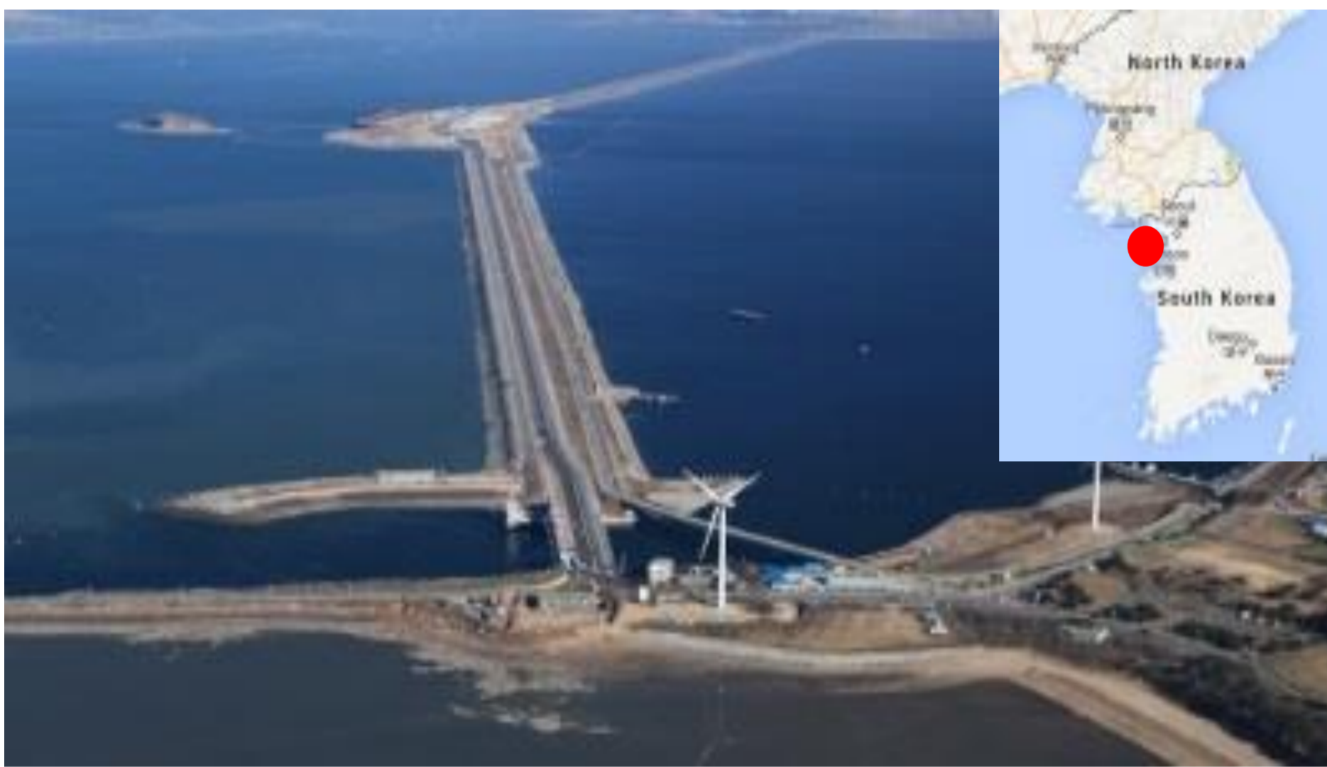
Fig. 1. Site of Sihwa microgrid system.
