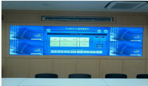
KMEG LOC @ Bldg. 220
