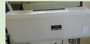
4 to 5 kW power conditioner for PV power generation
