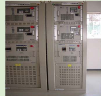
20kW Inverter type generator (simulates PV, FC, etc. )
