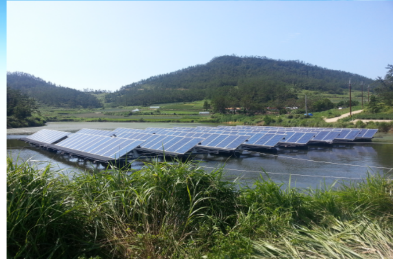
[Water Floating PV system : 48kW]
