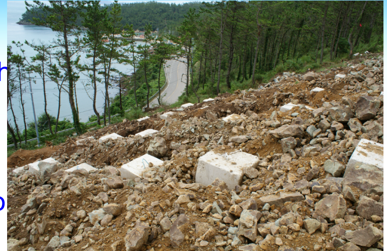
[Foudation of PV at the sloped site]
