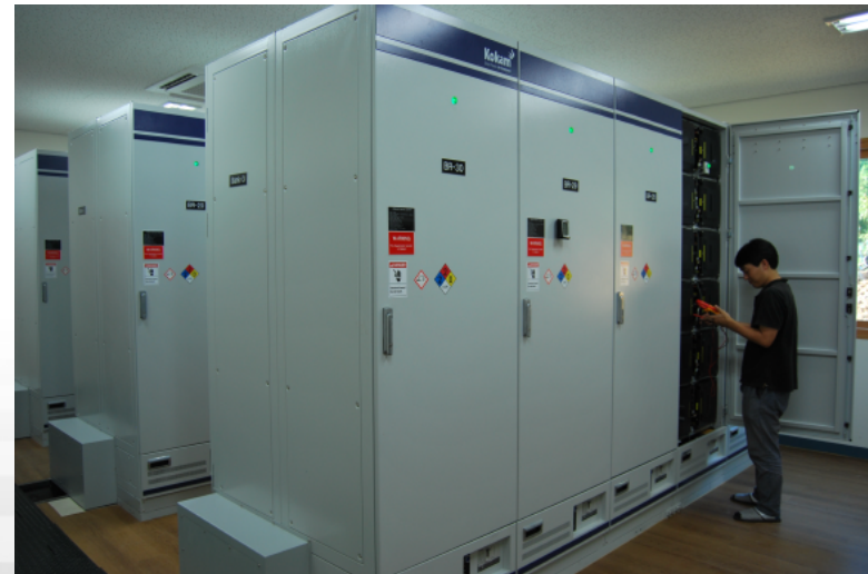
[Li-ion Battery : 3MWh]
