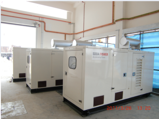
Diesel Generators
