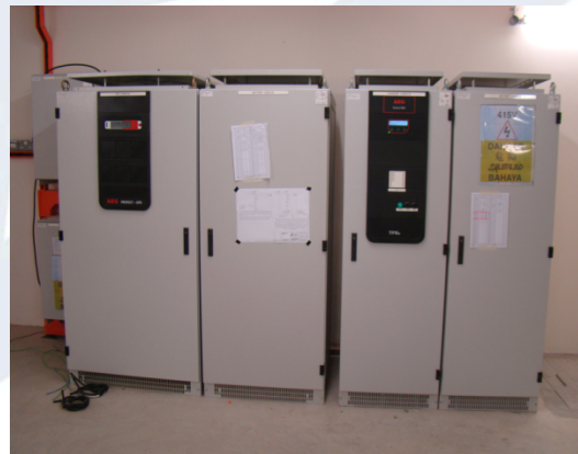
Uninterruptible Power Supply
